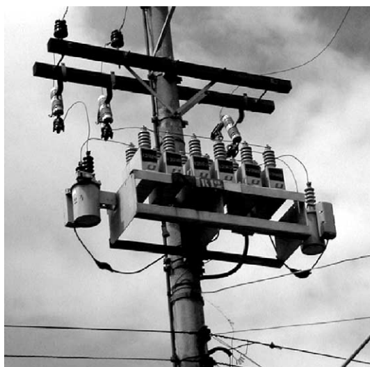
Fig. 3. Nine hundred kVAr CB at CPFL.
